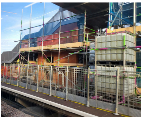
Pictured: Construction works at Newsham Station
